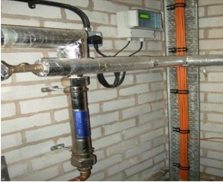
The lime scale prevention water treatment is supplied by a Sentinel Commercial KalGUARD system.
