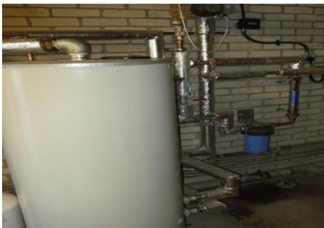
The system is mains fed, unvented hot water, feeding a 250 litre calorifier which holds the hot water for the Sports Hall demand.
