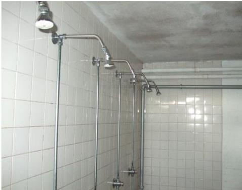
The showers are served by the calorifier and are routinely disinfected as per L8. Reports from site maintenance confirm that little or no lime scale cleaning of the shower head is required.
