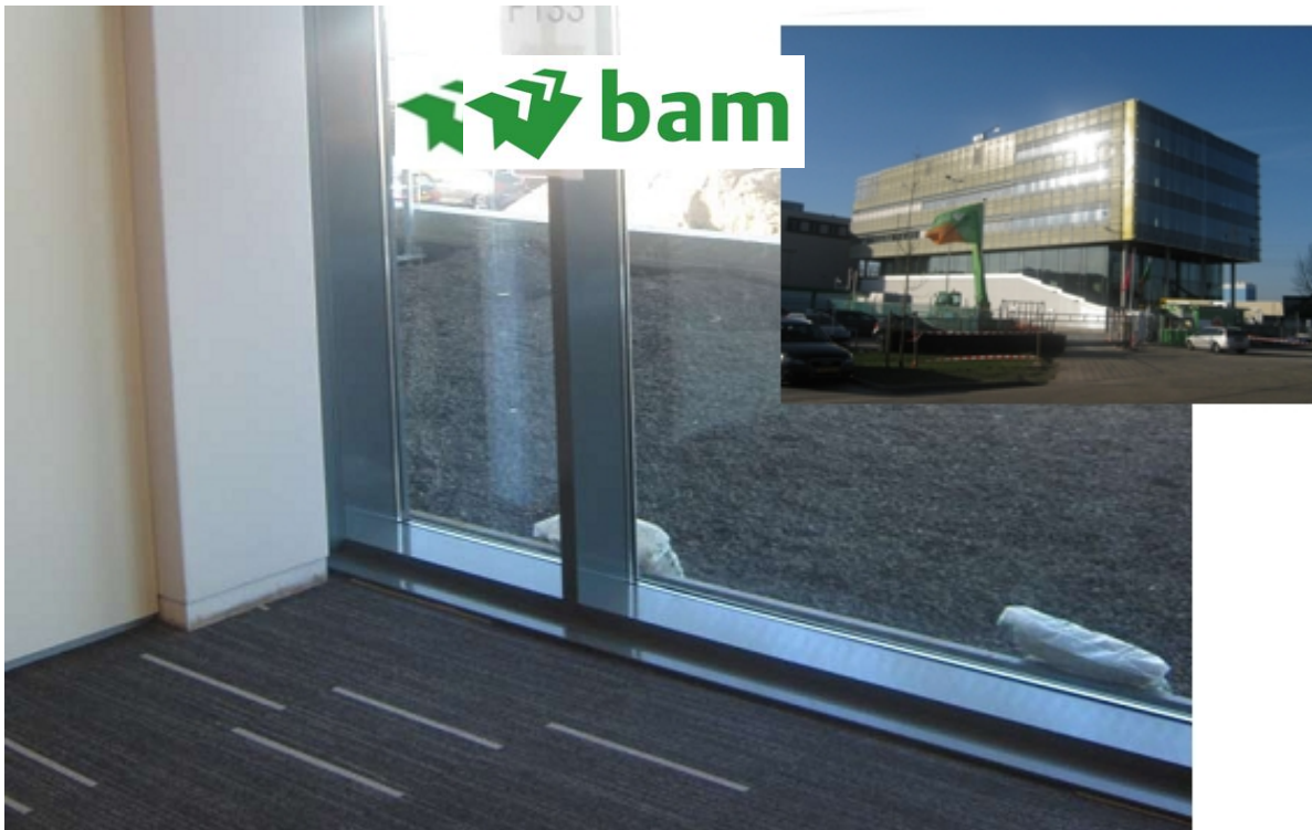
ThermaSkirt provides the heating and skirting in one – here seen at floor level, & matching the window frames.
