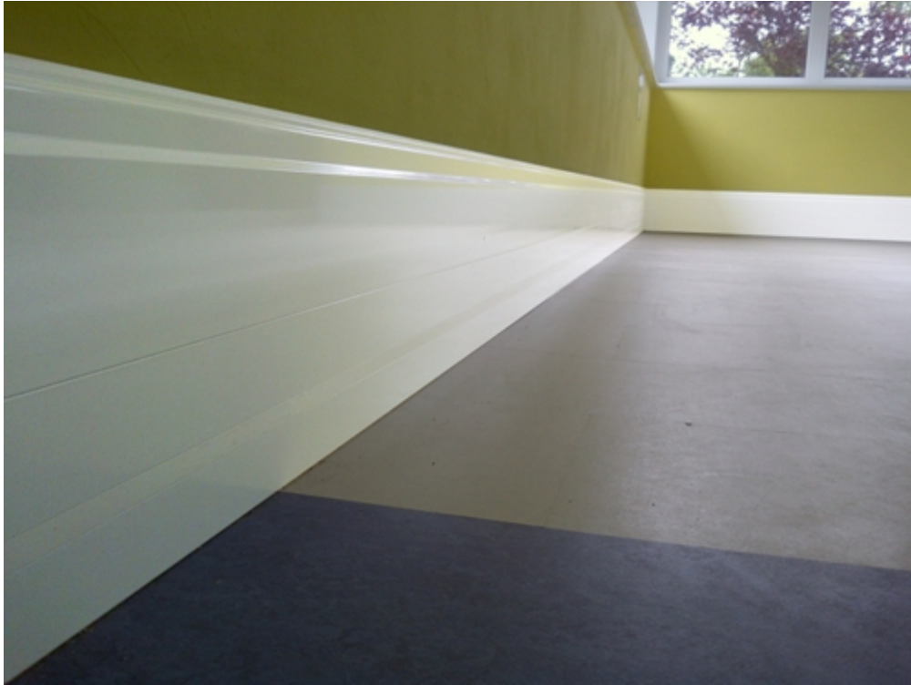
ThermaSkirt provides the heating and skirting in one – here seen in a double height profile.
