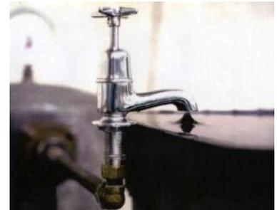
*This tap is sucking up potentially contaminated fluid because there is insufficient air gap*
