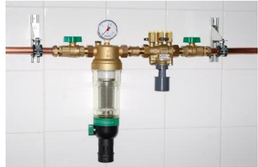
*Option F Assembly – with large capacity 100 micron strainer with semi-automatic back-flush facility. Ideal for laundry and high demand applications*
