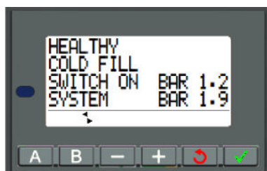
System Healthy – Cold Fill & System Pressures
