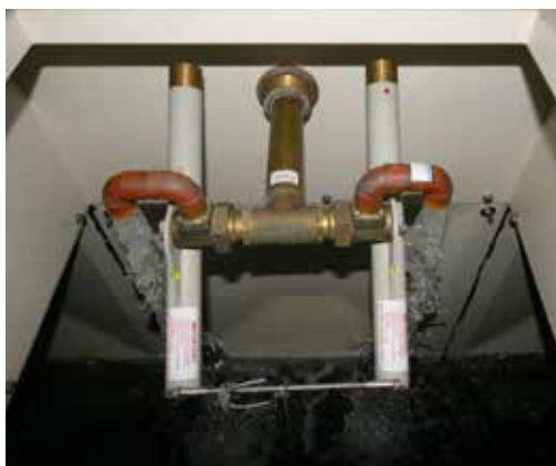
The delayed action of Aylesbury float valves delivers a positive fill to actively churn the water in the tank.
