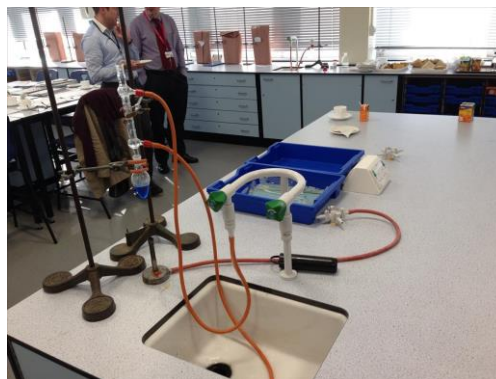
Fig 7: attaching laboratory equipment to lab tap compromises the "tap gap" – backflow protection is required e.g. supply from a storage cistern
