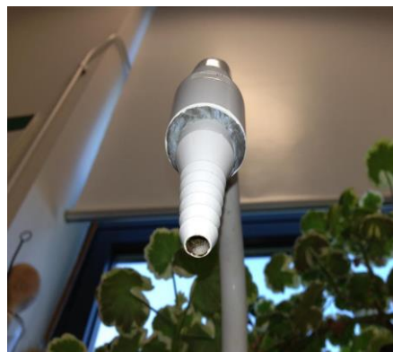
Fig 9: Any obstruction or interference with the air apertures, such as taping up or plugging, will eliminate the backflow protection placing the water supply at risk
