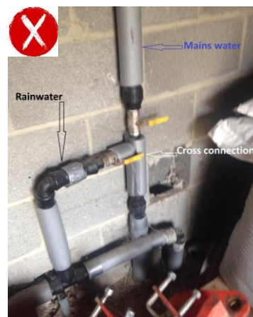
Fig 16: example of a cross connection between a rainwater and drinking water system
